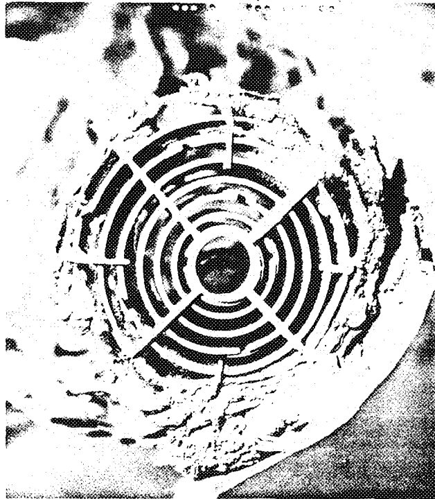
Fig. 86 - Upstream face of stage 4, cartridge 1060, cell 273
